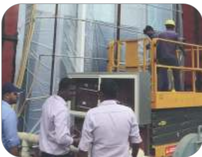
AIR INFILTRATION TEST
