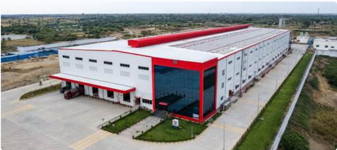
State-of-the-Art Plant: Supreme's modern extrusion facility in Kanpur, Uttar Pradesh, engineered on Industry 4.0 principles.
